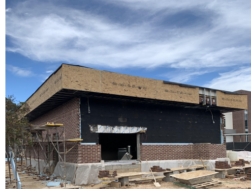
CSK- Concession Brick Install
